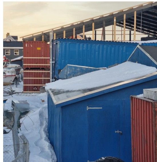
Slumping buildings in Ilulissat due to permafrost damage. Photo: Andreas Xion Magnussen Griis, Ilulissat
