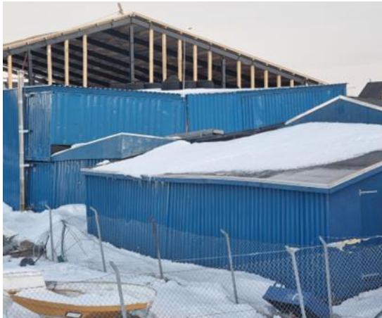
Slumping buildings in Ilulissat due to permafrost damage. Photo: Andreas Xion Magnussen Griis, Ilulissat
